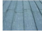
Lead cladding Used on rear roof end dormer
