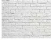
White painted brick - English bond Used on rear and side facades at B1 Level
